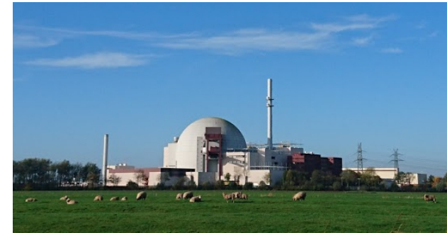
Nuclear power plant (Brokdorf, KBR)
