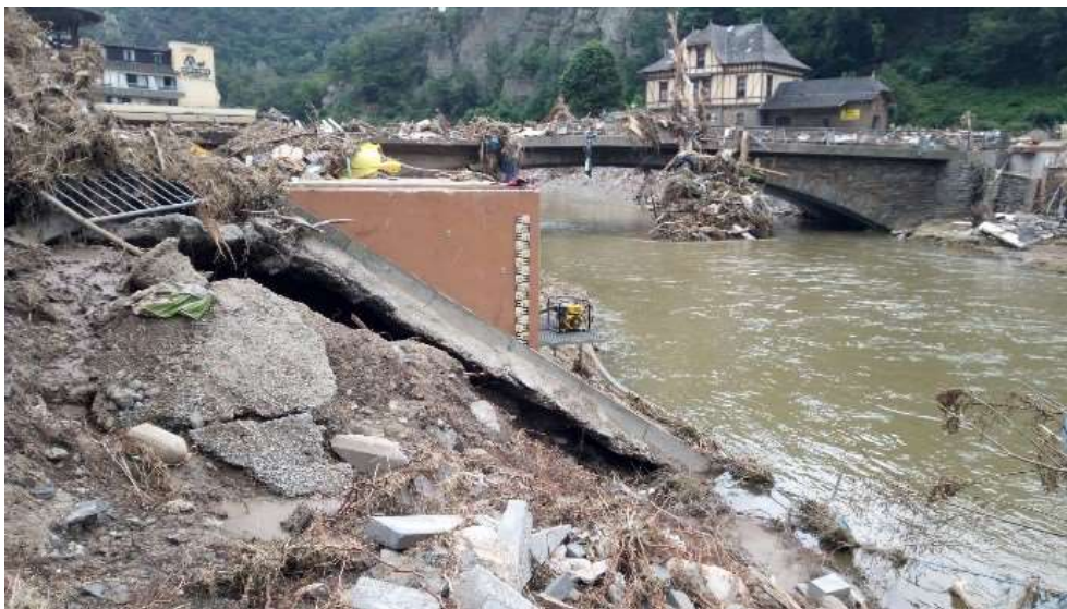
Figure 3: The Altenahr gauge before the flood in July 2021 ( top) and a few days after the flood (middle and bottom) ©SGD Nord
