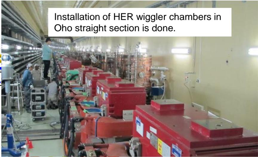
Installation of HER wiggler chambers in Oho straight section is done.
